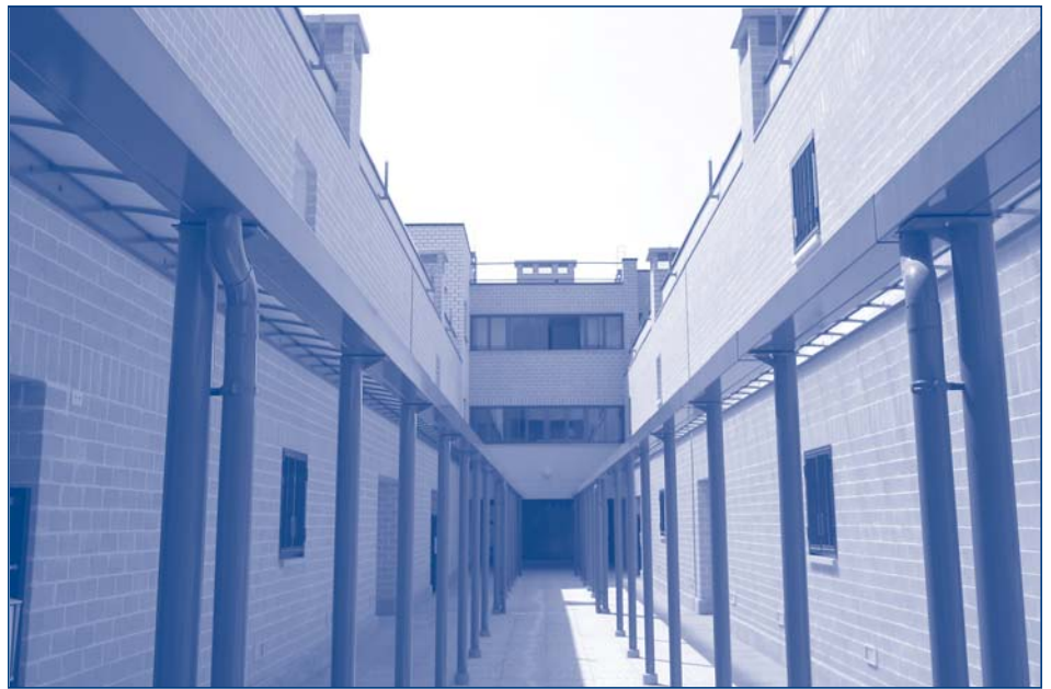
Co-op Dozza's Hygeia is separated into two adjoining buildings to give all the apartments terraces, sunlight, air circulation and plenty of windows. A passageway between the buildings connected by elevators allows for safe internal circulation.
