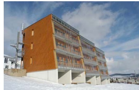
This residential building in the Czech Republic allows families to save considerable energy costs each month.
